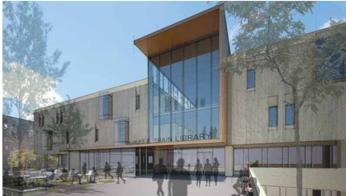
Over the next two years, a $7.5 million renovation of the Charles E. Shain Library will quadruple collaborative study spaces for students.
